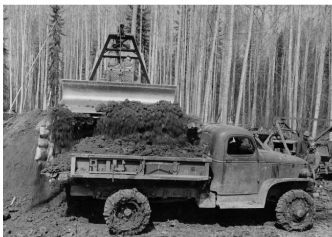
Figure 3: Dozer drifting loose soil into a 1940 Chevrolet 4x4 1-1/2 ton (1360 kg) capacity dump truck. It is hauling fill for an airport access road in May 1942 (Source: US NARA).
