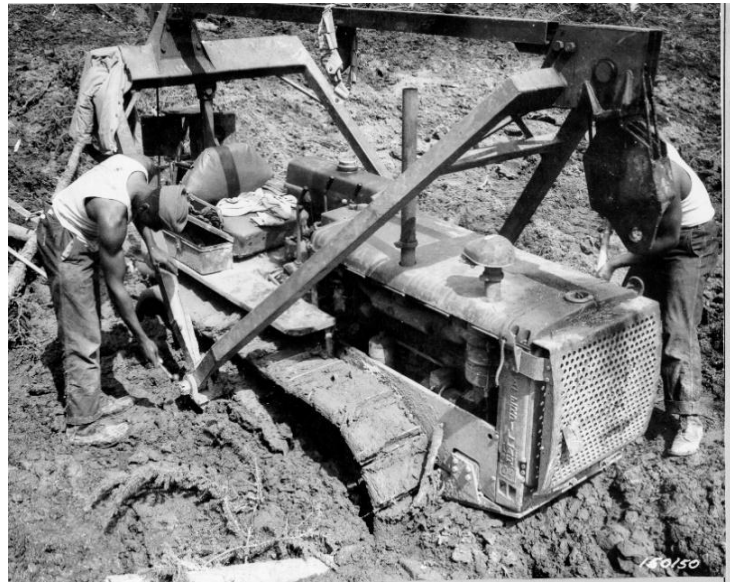
Figure 13: Tracked dozer swallowed up by a muskeg hole. Muskegs sometimes appeared to "swallow" the heavier equipment, then exhibiting thixotropy, when the silty mud mixture "sets up." (Unknown date. Source: US NARA).
